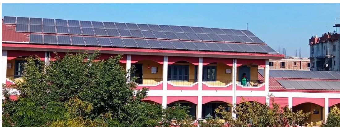
Fig. 6: Roof top solar panel, K.C. Das Commerce College
